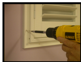
Only secure one screw into the bottom left frame.
