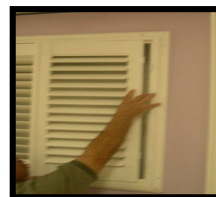
Insert panel into position.
