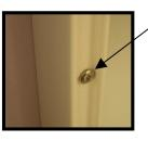
**Tip:** It is best tightening round head screw and counter sinking screw if possible to allow inserts to properly snap into frame.
