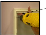
Only secure <u>one</u> screw into the top left frame.
